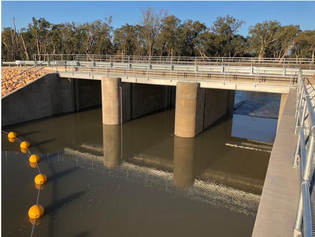
Figure 1: 'The Splash' environmental regulator on the Katarapko floodplain in operation (Source: DEW)
